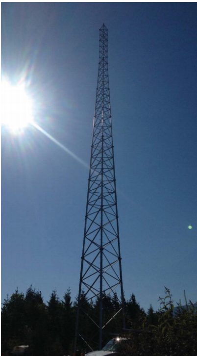
Parallel Infrastructure's newly stacked tower in Skagit County, Washington.
